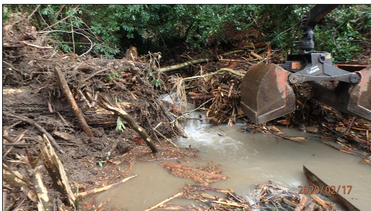
Photo provided by RCT's Flood Risk Management team showing woody debris on the debris screen of the Pentre Road culvert inlet on the 17 th February 2020.
