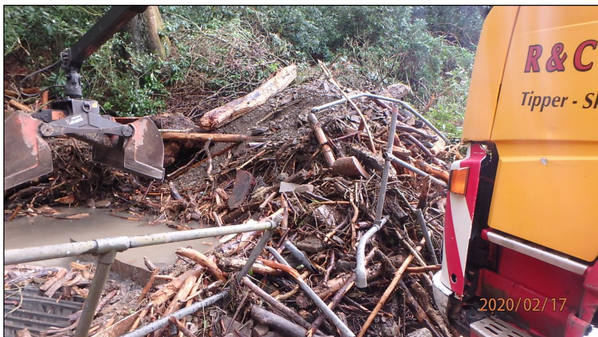
Figure 16: Photo looking across the Pentre Road culvert inlet, showing significant material collected during Storm Dennis (17/02/2020)
