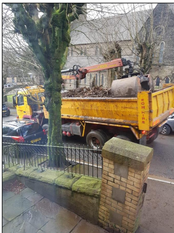
Figure 18: Photo showing woody debris being transported away from the Pentre Road culvert inlet during emergency clearance works (17/02/2020) (image provided by resident)
