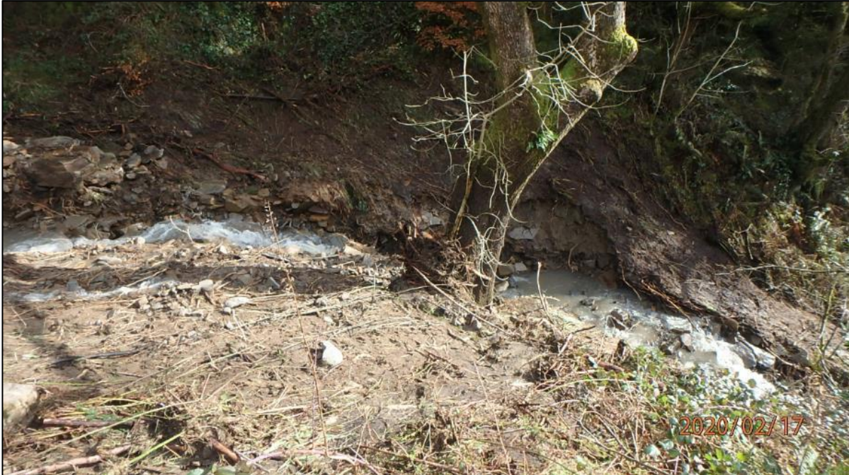
Figure 23: Photo of minor scour to the embankments of the Nant y Pentre watercourse in the upper catchment of Pentre (17/02/2020)
