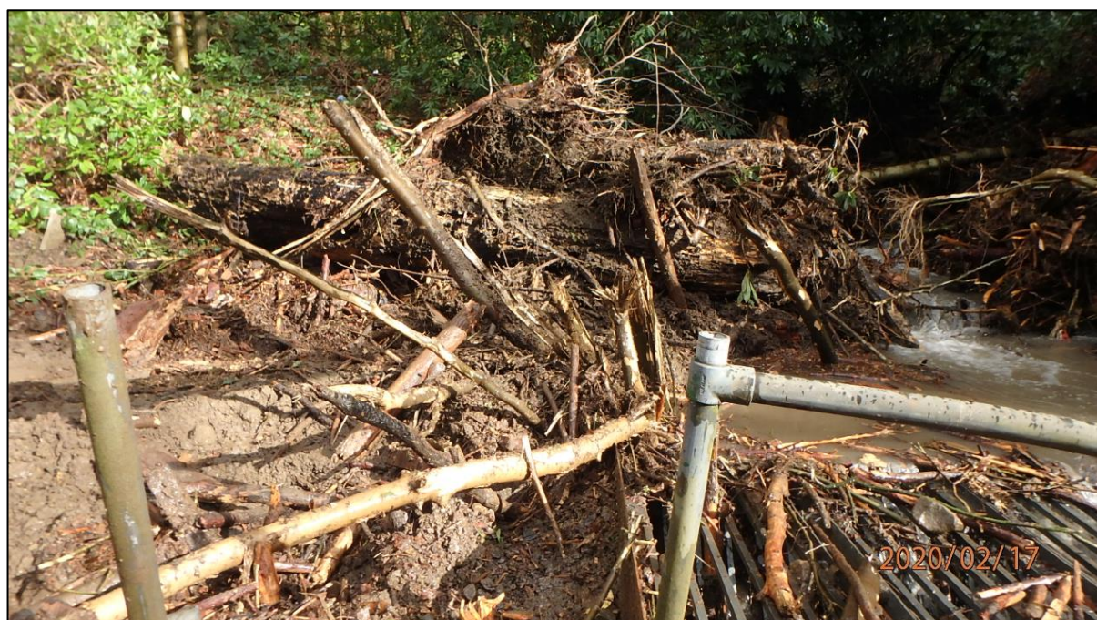
Figure 17: Photo of Pentre Road culvert inlet showing significant woody debris deposition (17/02/2020)
