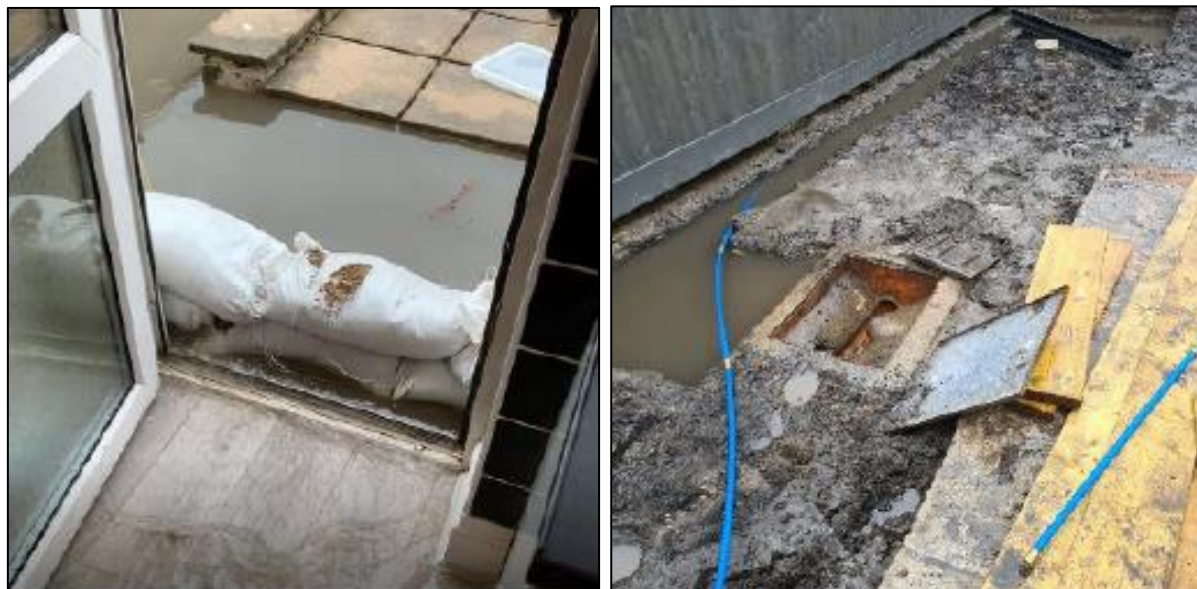
Figure 12: Water entering the Queen Street property via the back door (left) and location of surcharging manhole at Treharne Street, causing internal flooding to three properties (right)
