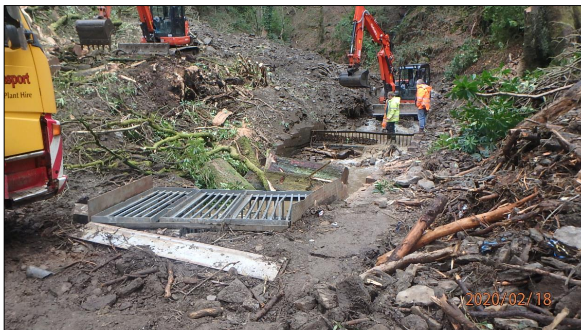
Photo provided by RCT's Flood Risk Management team of the Pentre Road culvert inlet and channel following emergency clearing works on 18 th February 2020.
