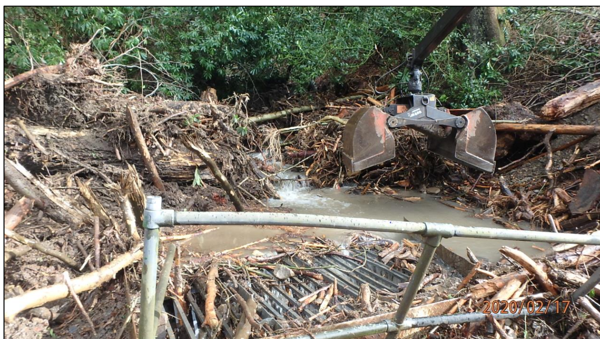
Figure 15: Photo of Pentre Road culvert inlet during works to remove deposited material post Storm Dennis (17/02/2020)
