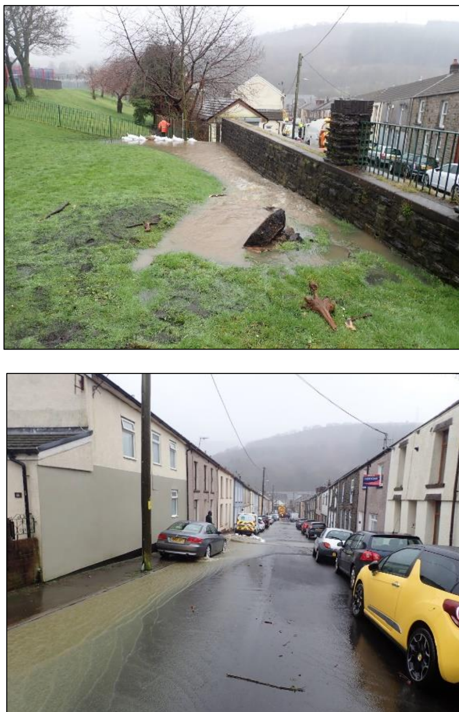
Figure 9: Surcharging manhole within Pleasant Street Park (top) and flow path down Pleasant Street (bottom) taken by RCT's FRM team on 20 th February 2020
