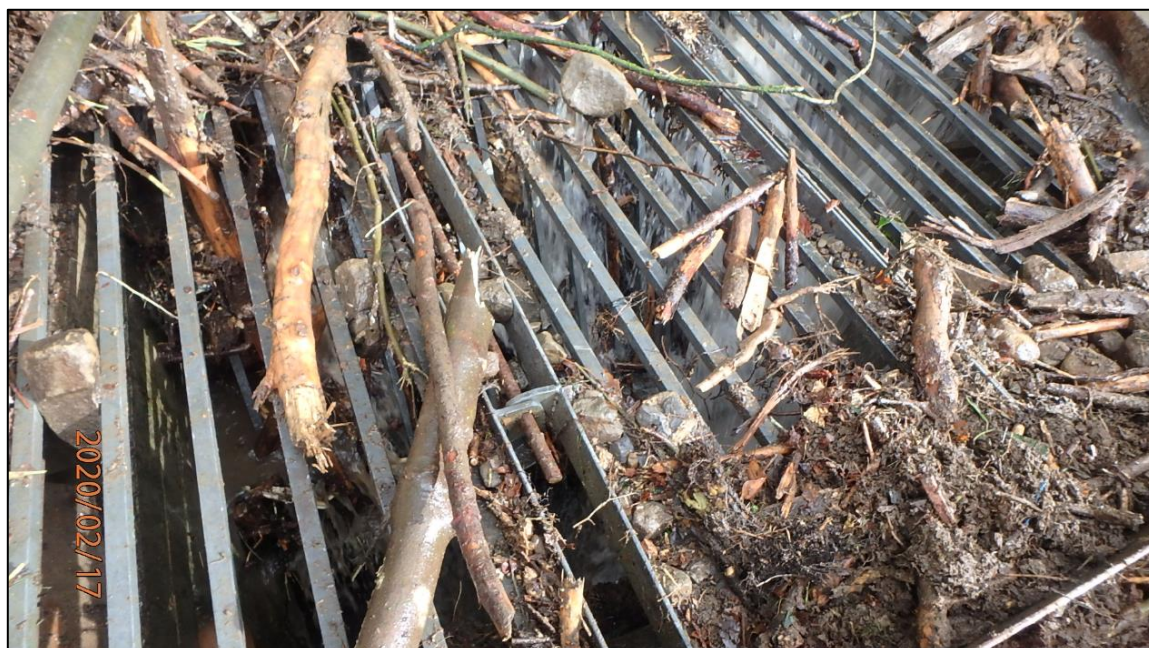
Photo provided by RCT's Flood Risk Management team showing woody debris in the Nant y Pentre channel and at the culvert inlet on 17 th February 2020.
