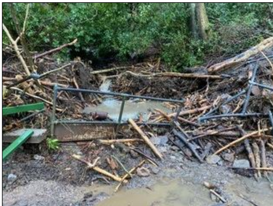
Figure 14: Photo of Pentre Road culvert inlet captured by RCT's Highways and Streetcare Depot immediately after the storm event (16/02/2020)
