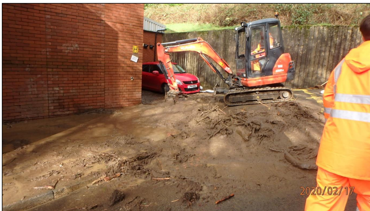
Photo provided by RCT's Flood Risk Management team showing woody debris and mud being cleared to the rear Pentre Road Care Home on the 17 th February 2020 (situated directly downstream of the Pentre Road culvert inlet).
