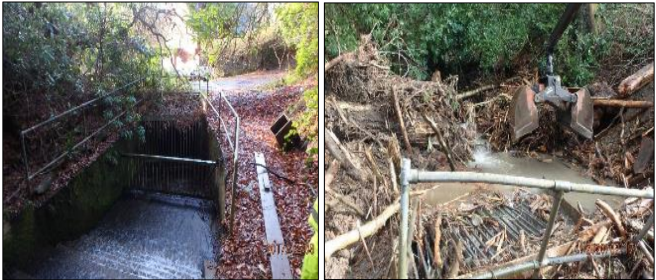
Figure 15: Pentre Road culvert inlet pre (left) & post Storm Dennis (right) showing evidence of significant blockage to the inlet
