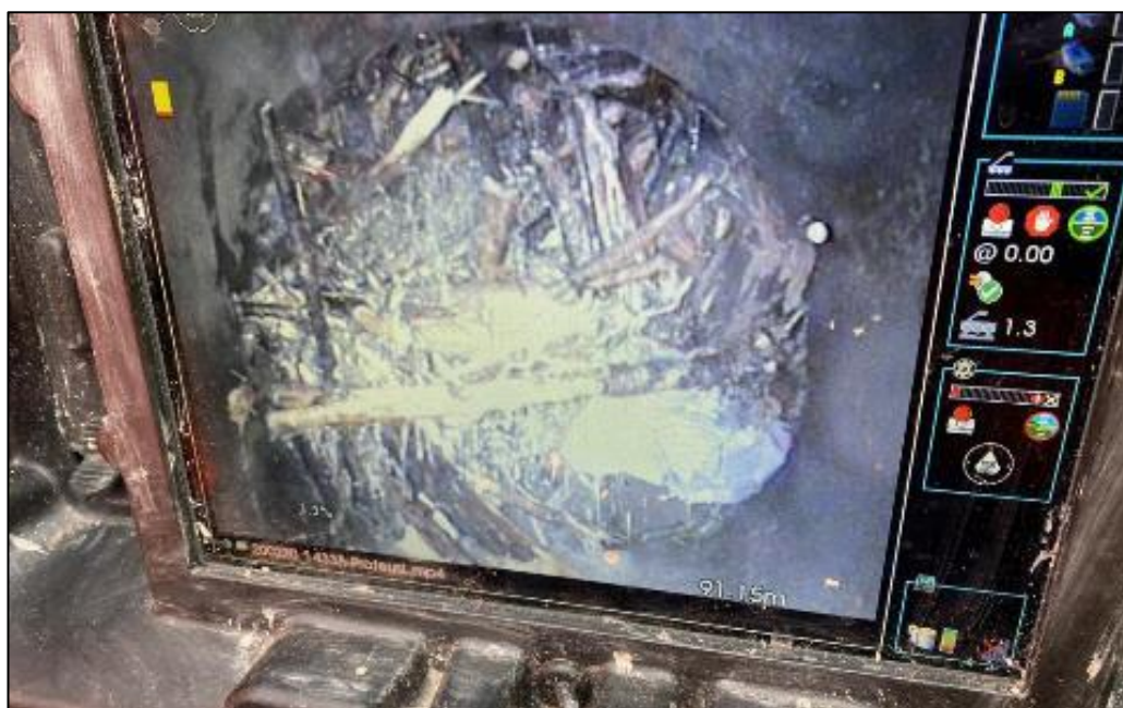
Figure 19: Photo showing full-bore blockage of the Pentre Road network downstream of Pleasant Street Park manhole
