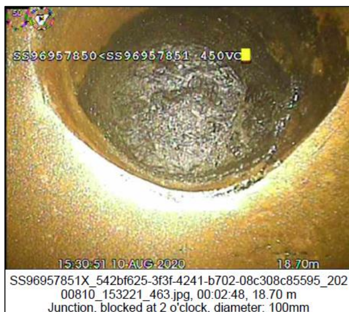
Figure 26: CCTV footage showing blockage on Lewis Street highway drainage network
